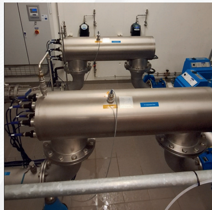
Figure 3 A UV disinfection water treatment system
